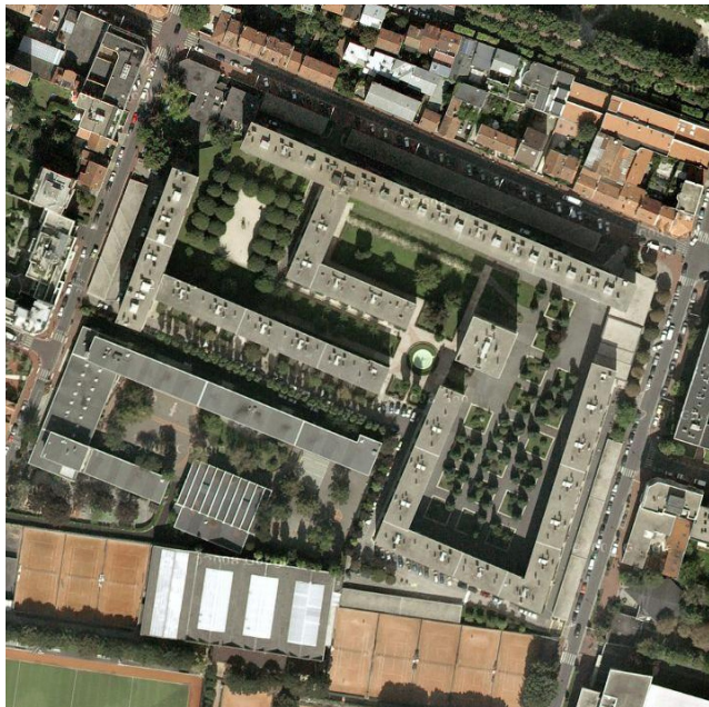
Avenue Fort, 92120 Montrouge, France
